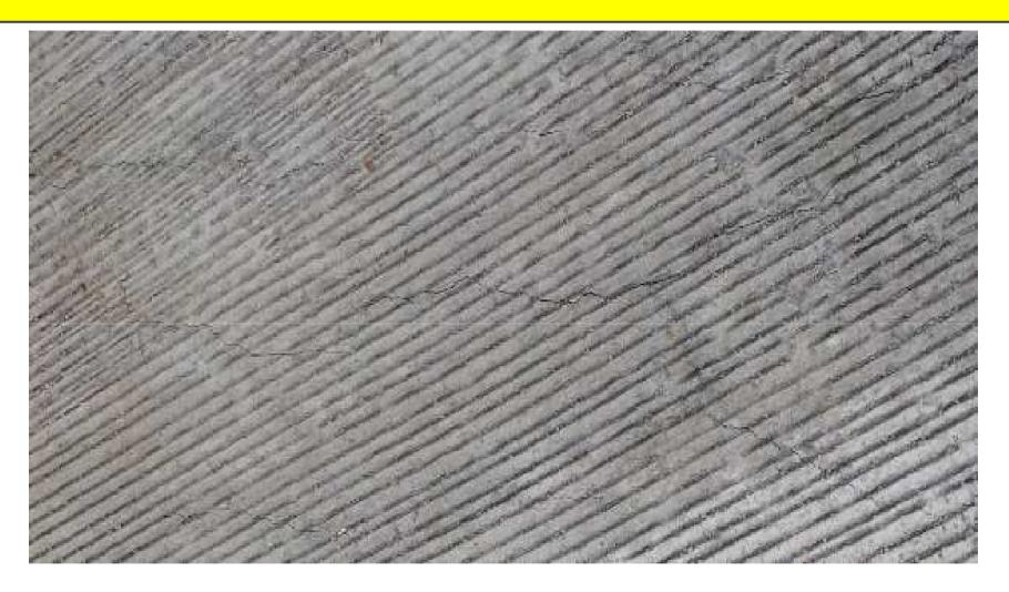
Plastic shrinkage cracking on surface of Concrete Road (with silica fume) - no bleed water and no early curing!
