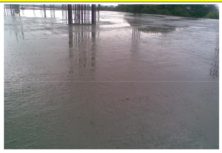
Bleeding Water comes upto slab surface immediately after casting
