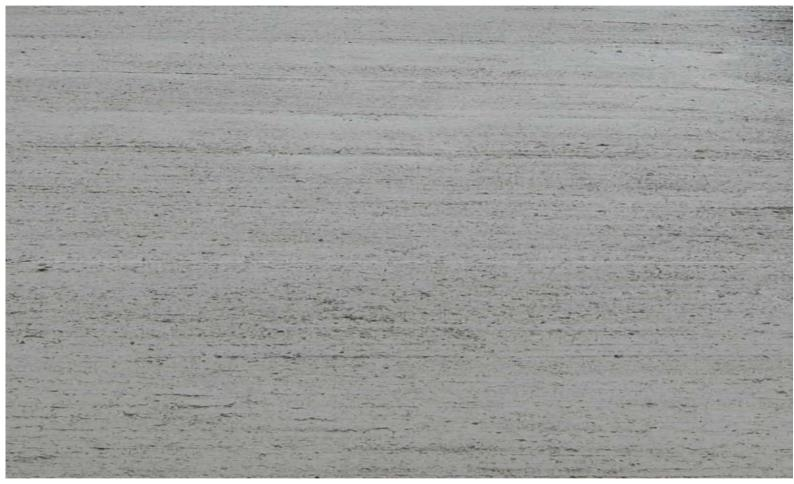
Surface can become dry/sheen-less when Concrete is still plastic within few minutes to few hours depending on the atmospheric conditions and mix used
