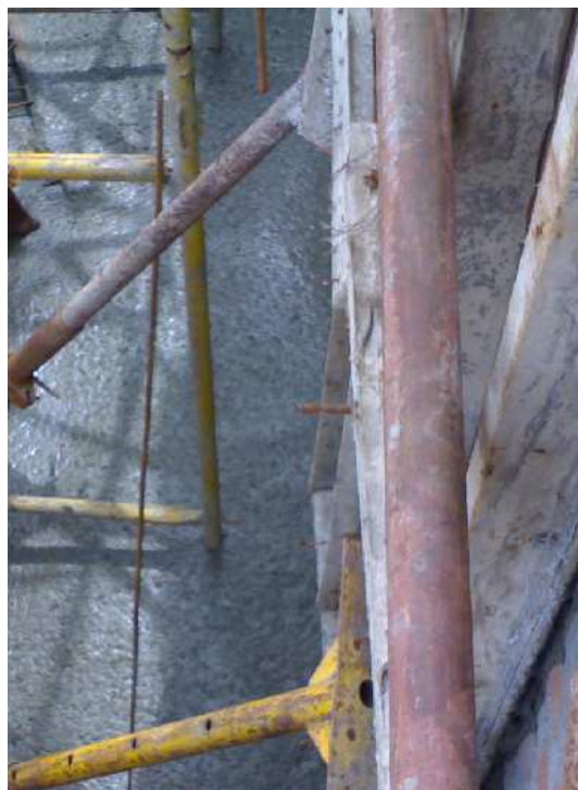
SCC fallen from a height of 8 feet due to inadequate support to form work – yet homogeneous
