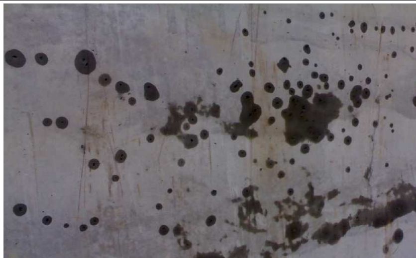
Blow holes on SCC surface – not a structural issue but an appearance concern
