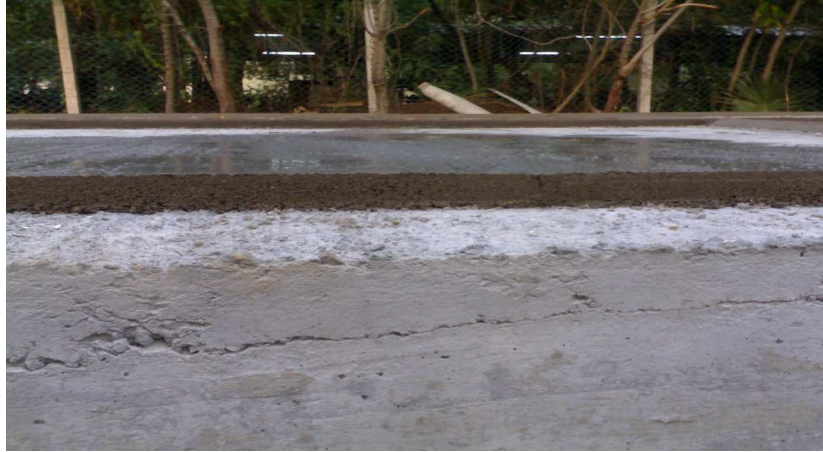
Cold Joint in SCC (Floor Slab element)
